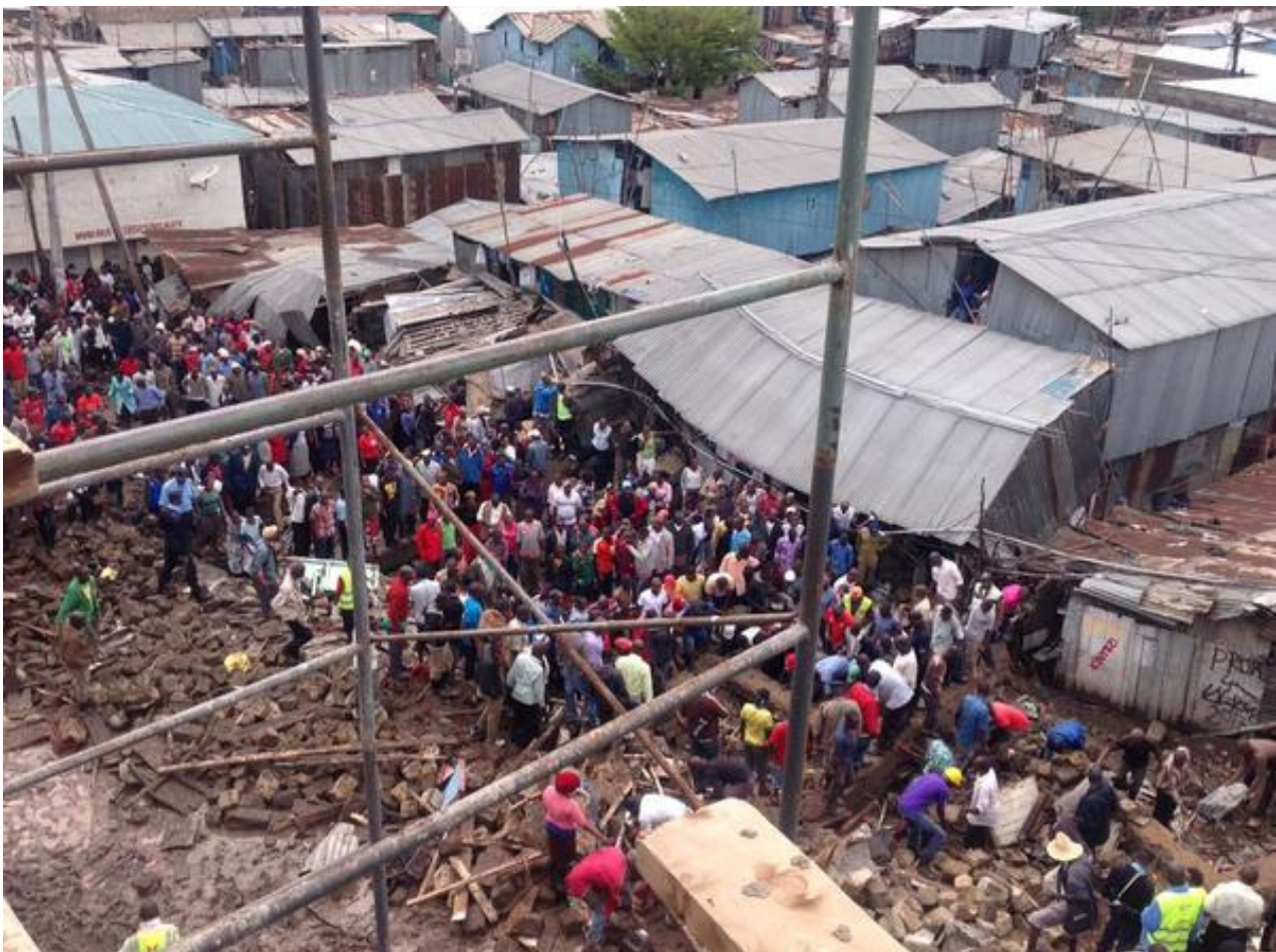
Image 2: Building collapse in Nairobi after heavy rains (Kenya Red Cross 2015)
