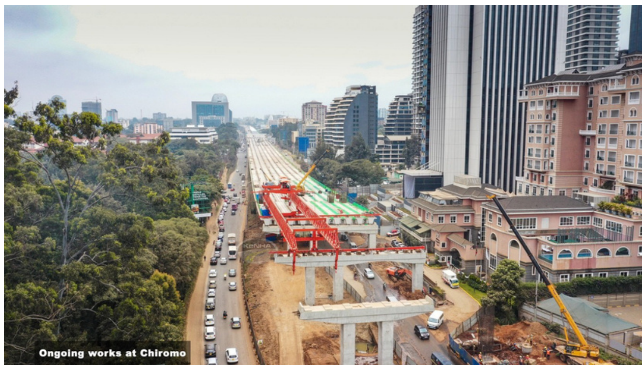
Image 1: Construction of the Nairobi expressway (Kenya National Highway Authority, 2021)
