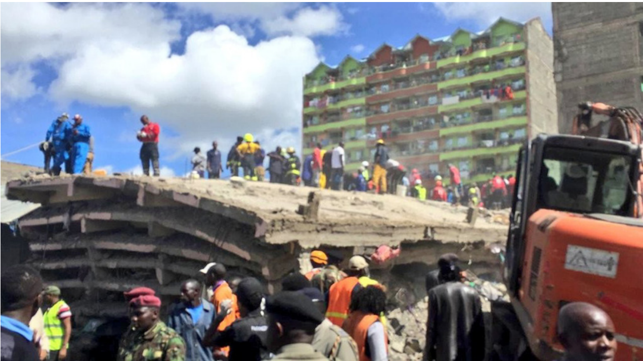
Image 3: A building that collapsed due to alleged flooding (Kenya Red Cross, 2019)
