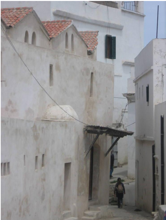
Image 1: Algeria's traditional windows, which make homes more private and block more sunlight (UNESCO/Hana Aouak)
