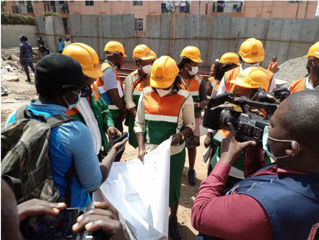
Image 1: Officials from the National Building Review Board halt construction at a site where workers are building a different structure than indicated in approved plans (NBRB 2021)
