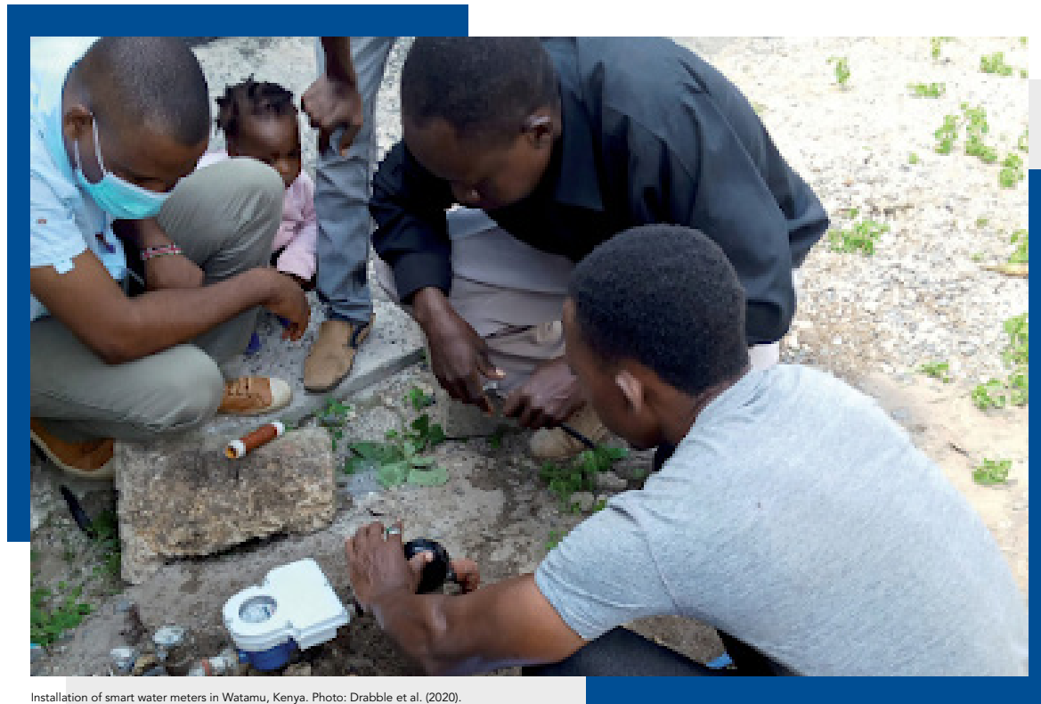
Installation of smart water meters in Watamu, Kenya. Photo: Drabble et al. (2020).
